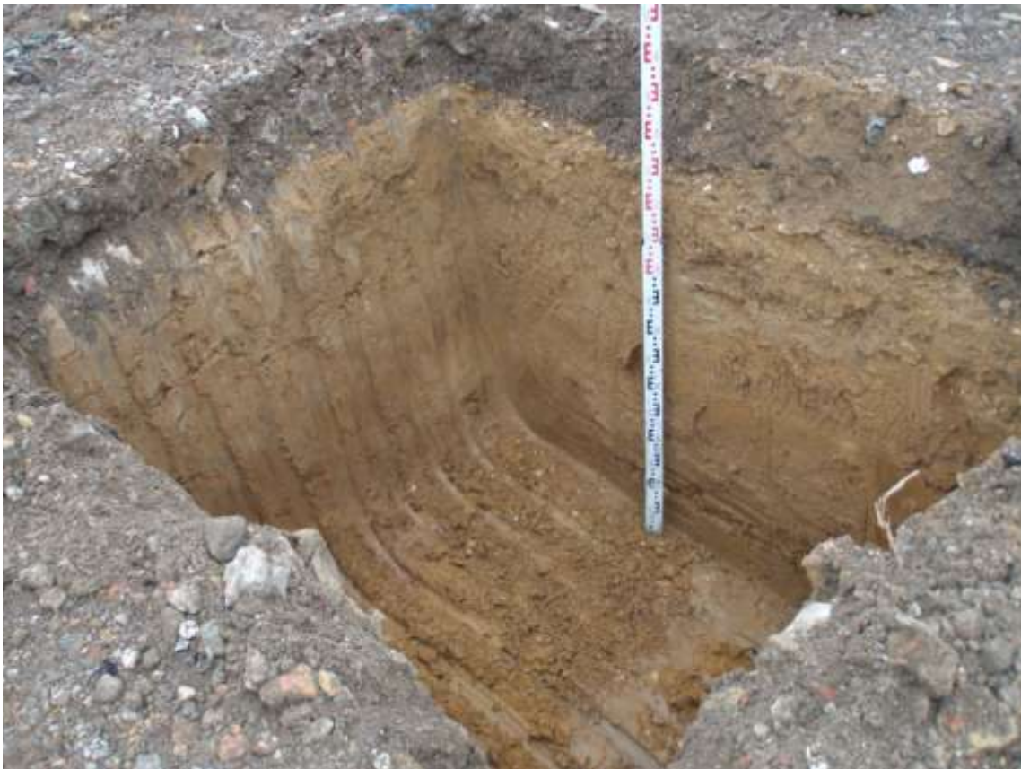
Plate 3. View of post pad trenching (looking NE)
