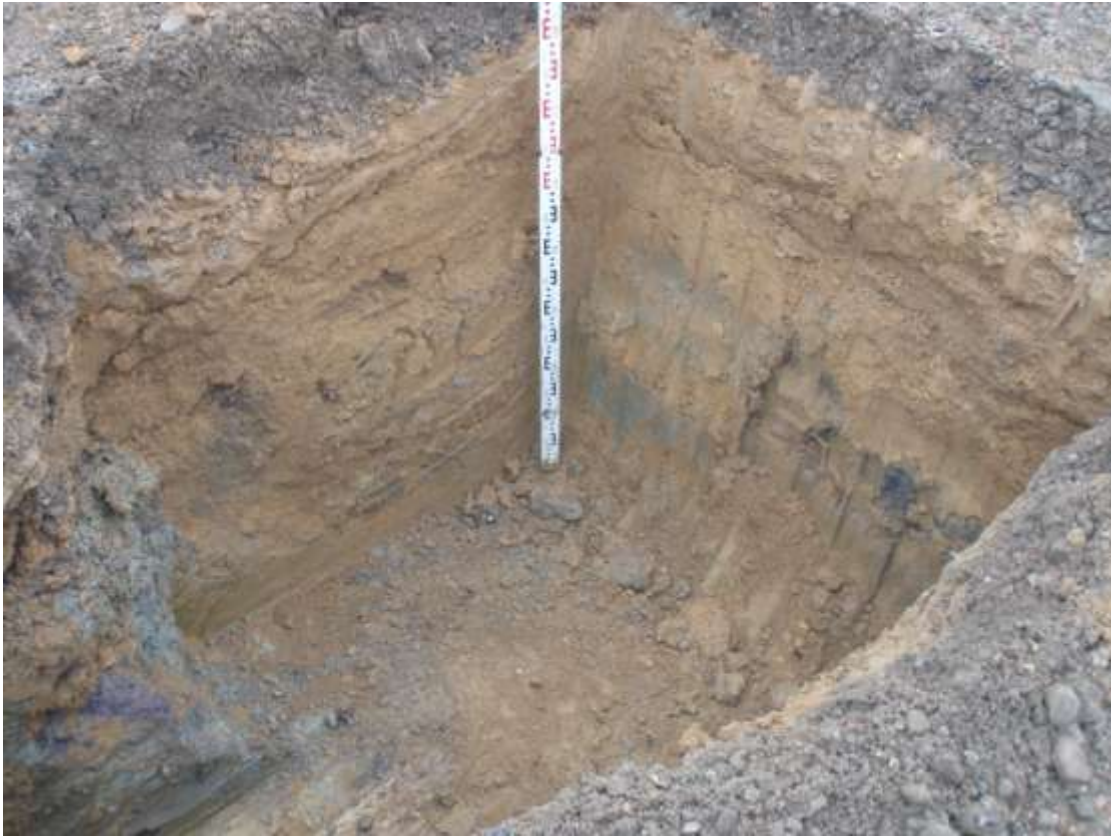
Plate 6. View of the post pad trenches (looking NW)
