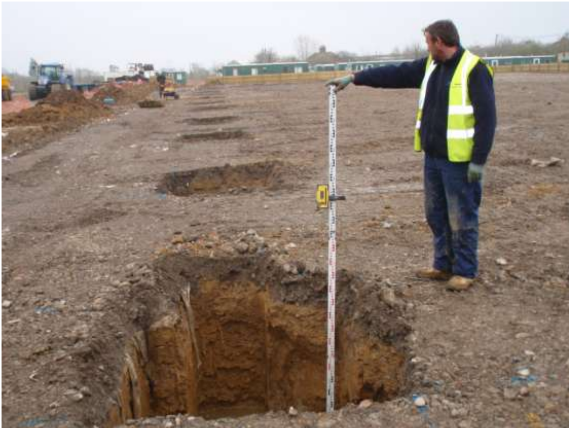
Plate 5. View of the post pad trenches (looking NW)
