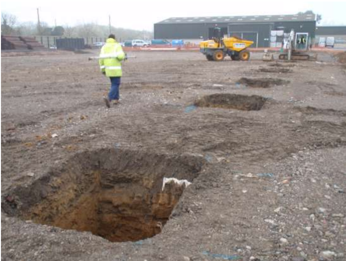
Plate 7. View of the post pad trenches (looking NW)
