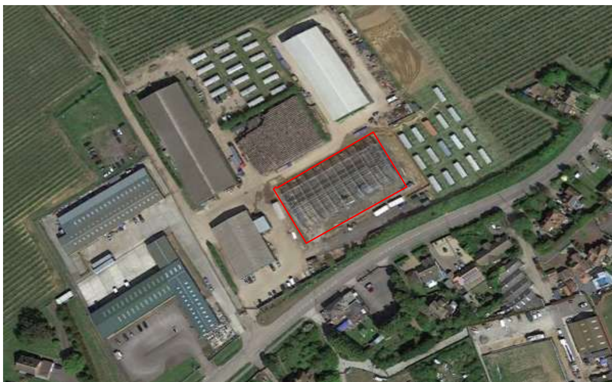
Plate 1. Aerial view of site (red line area) showing the site being developed and area watched
